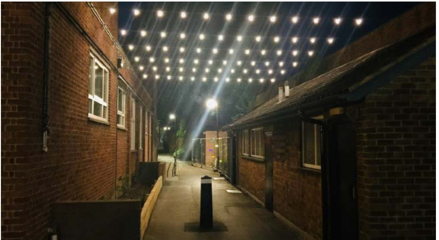
Light installation for safety and interest
