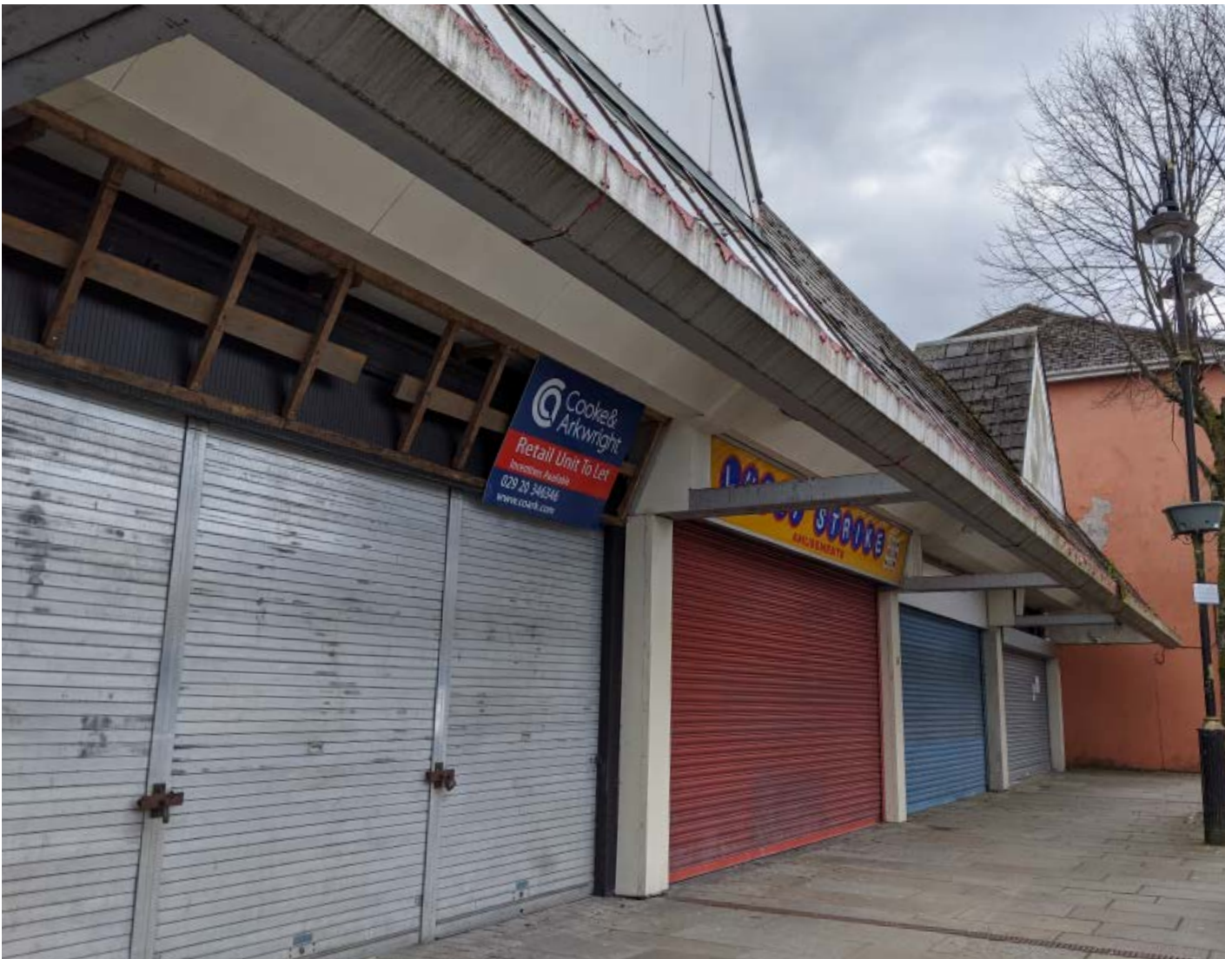
Vacant units to Gwent Shopping Centre Facing Commercial Street
